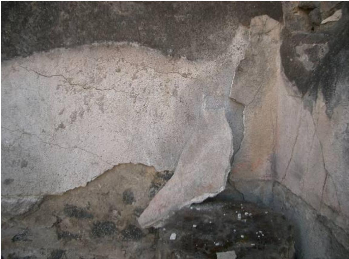
Fig.18. Above to the left: Edifice of Eumachia, space 222. Detaching wall plaster.
