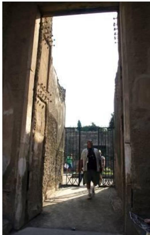
Fig.2. Via dei Soprastanti, different building constructions; to the left an area of *opus incertum*, in front to the right a technique of the Roman period with use of baked brick, *opus testaceum*.
